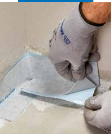
Application of Mapeband SA in corners
