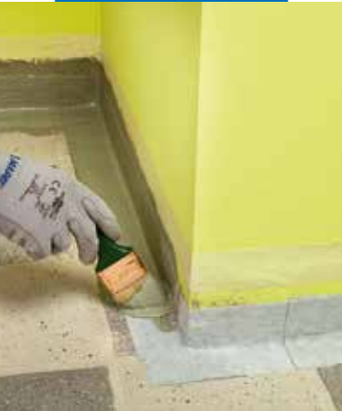
Application of Mapeband SA on a screed
