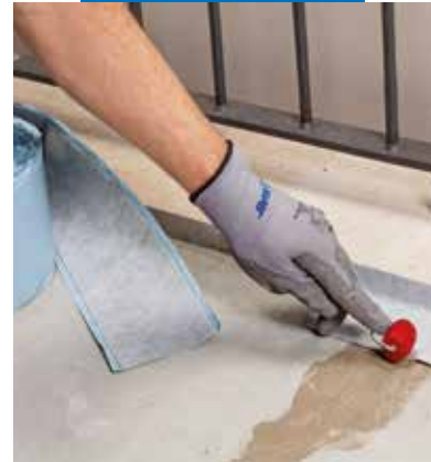
Application of Mapeband SA around edges
